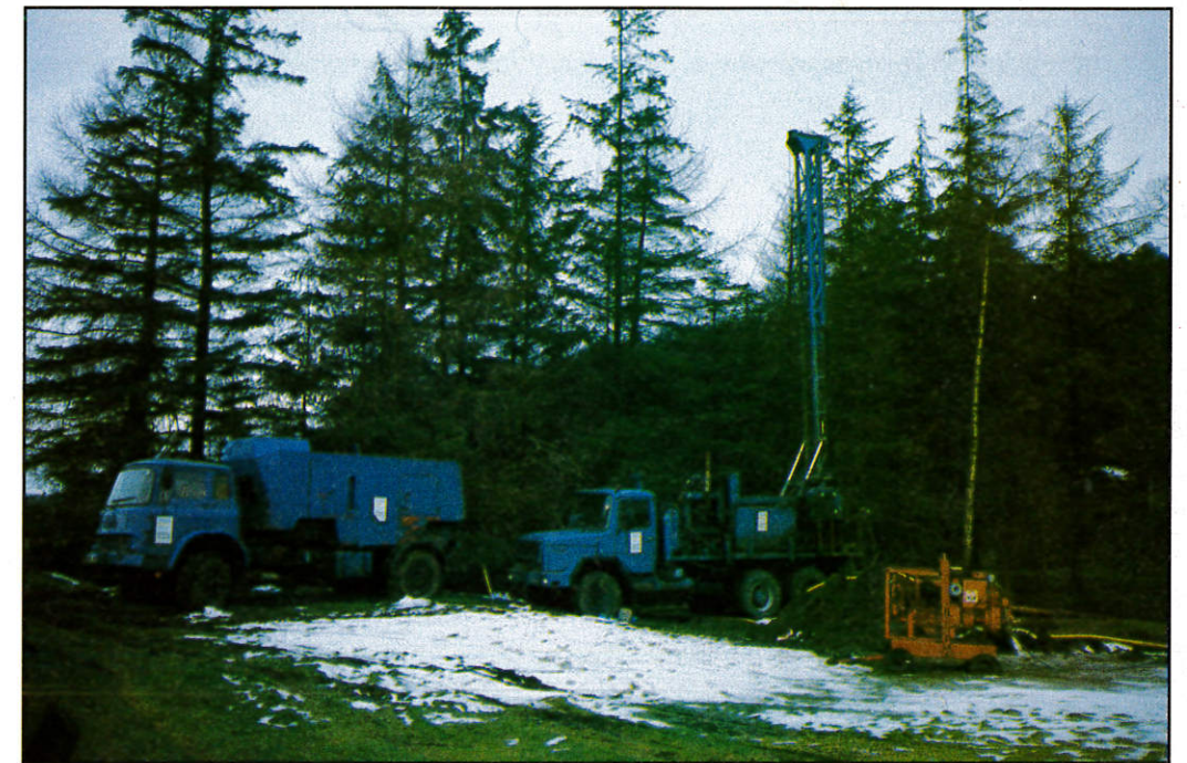
At work on a borehole at Ilkley Golf Club.
