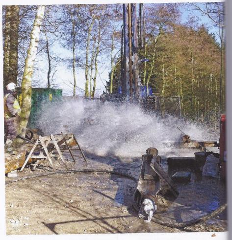
aquifer (water bearing rock), cased to maintain the integrity of the hole and delivered approximately 10m3 per hour, easily meeting the site's demand for water. The pumping plant was installed to deliver the water and a water sample for analysis was taken, with the water being suitable for use straight out of the ground. Occasionally this isn't the case but even with water treatment the economics still makes sense."
